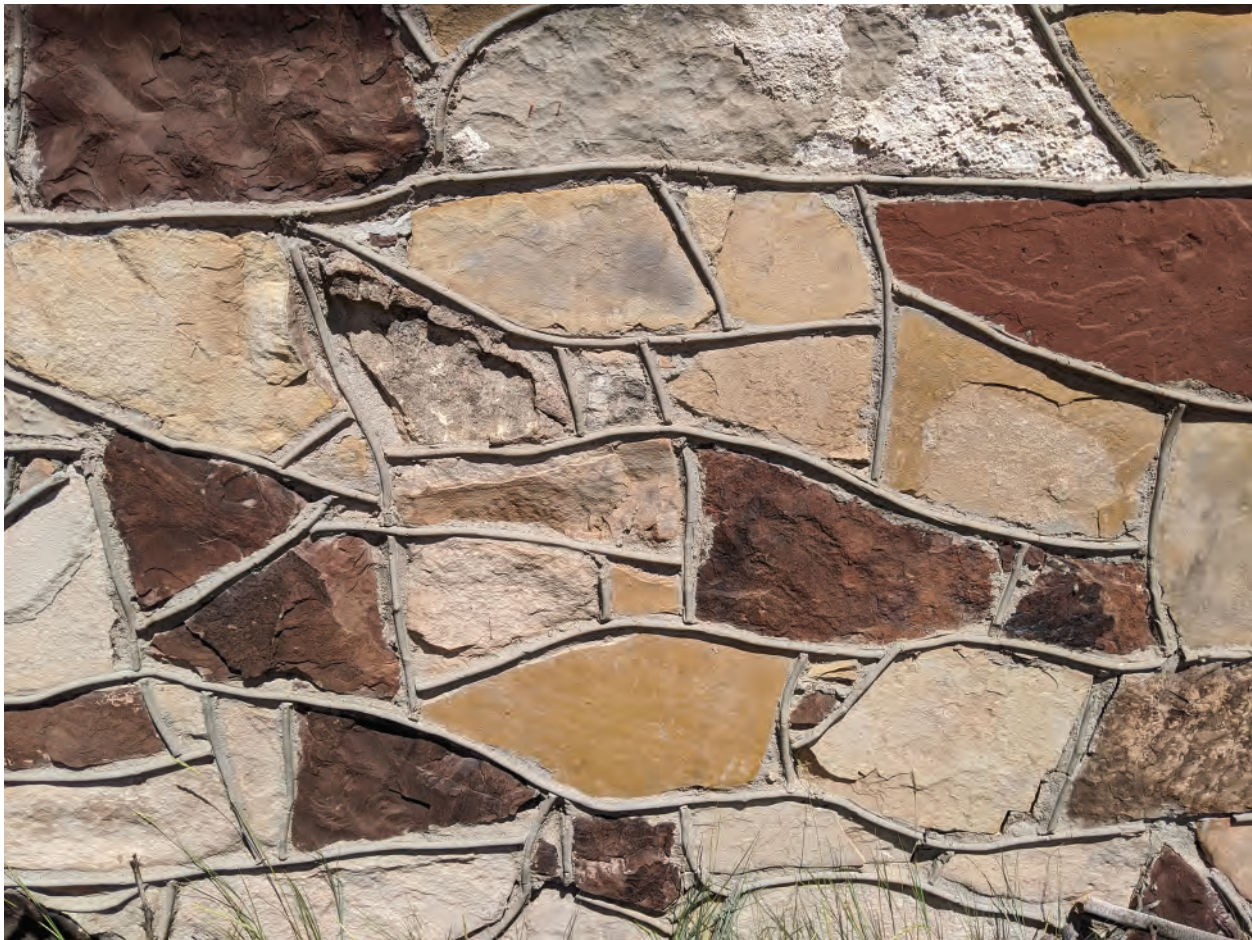
Figure 3. Raised mortar in giraffe style, Mountainair, New Mexico.
