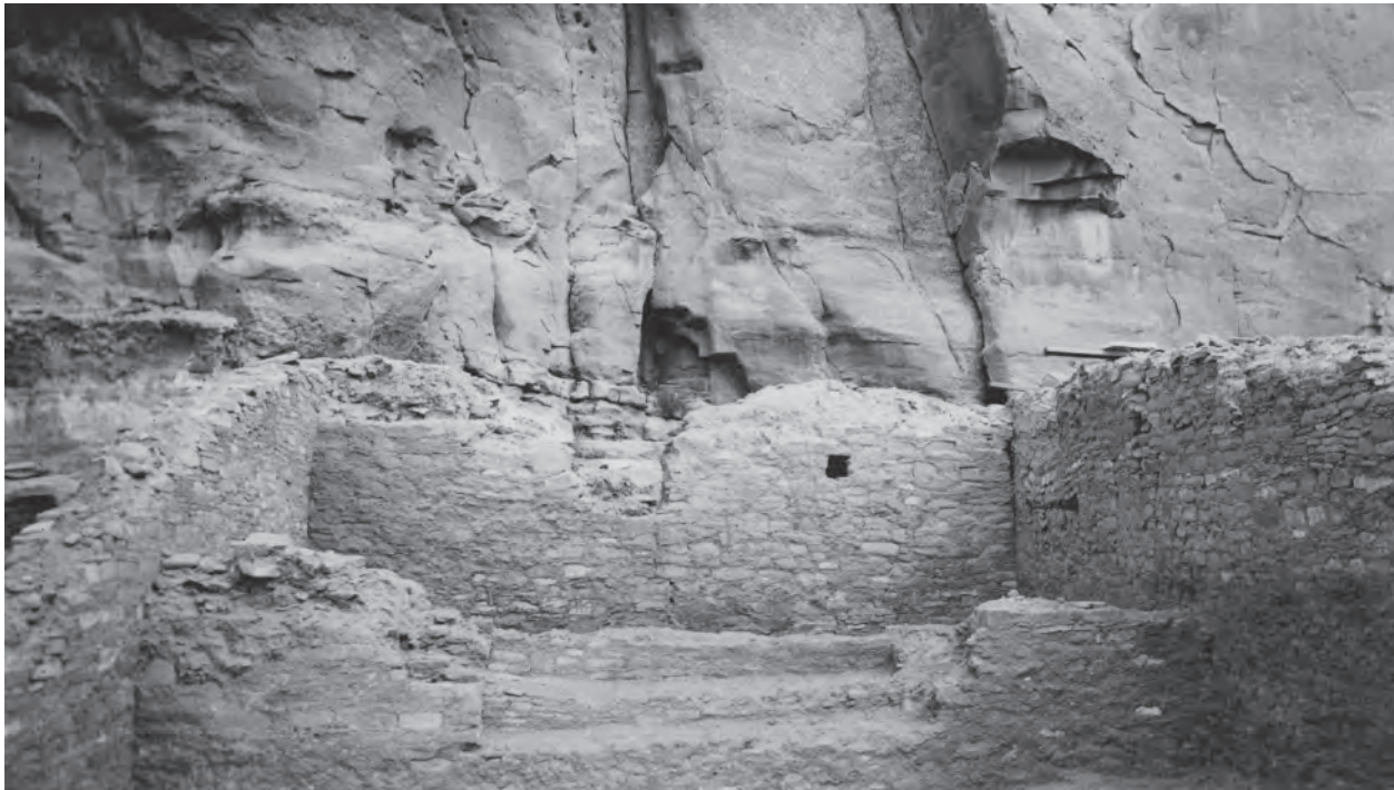
Figure 7. View of the north wall of Room 8 as published by Woods (1934:Plate IV, Figure 2). Note the major portion of a doorway and damage on the west side of the north wall has been filled in. (Courtesy of the Palace of the Governors Photo Archive, Negative No. 81277.)
