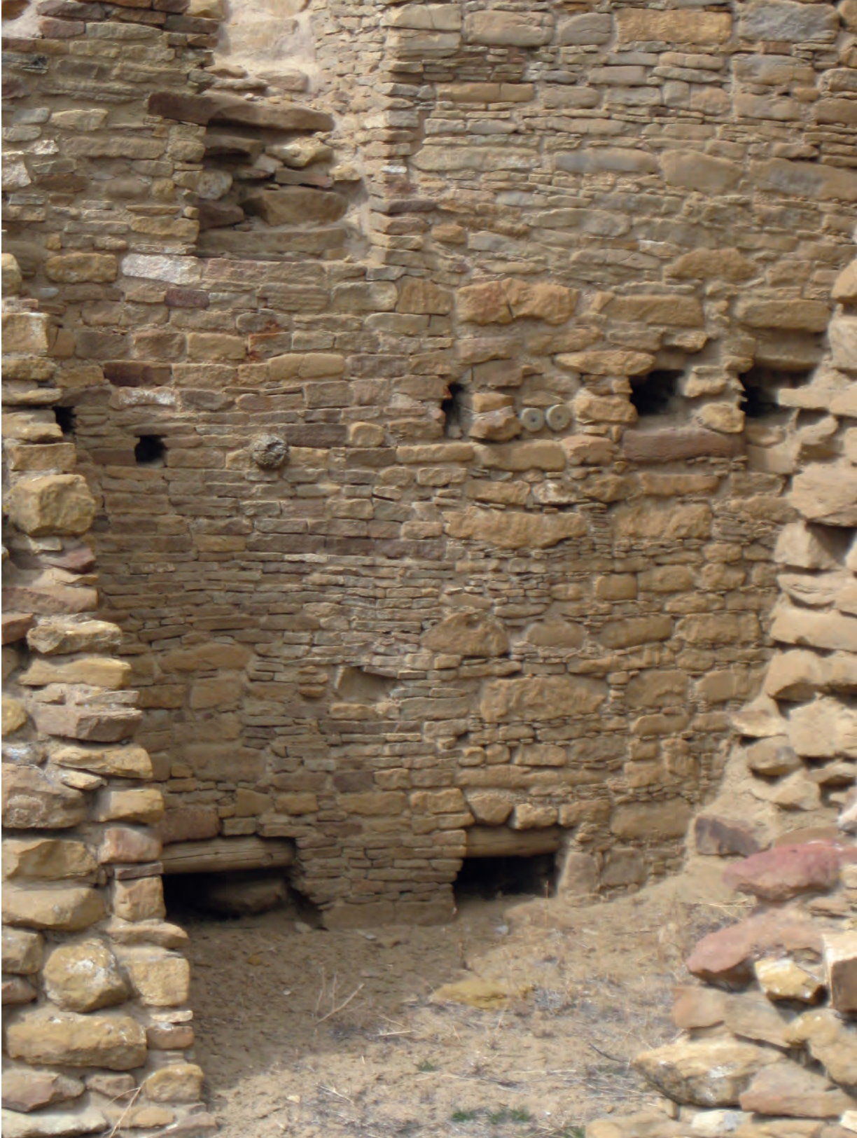
Figure 10. Photo of exterior east wall of Room 23/33 taken in 2020. Note the latilla hole (No. 7121) visible in Figure 9 has been filled in. Photograph by Richard Voorhees.
